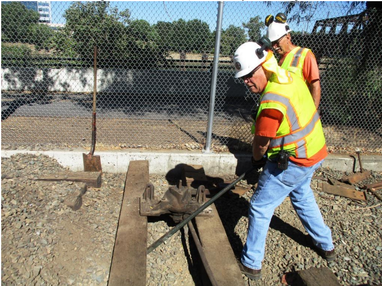
Bill uses a lining-bar to "bar over" the head-block
