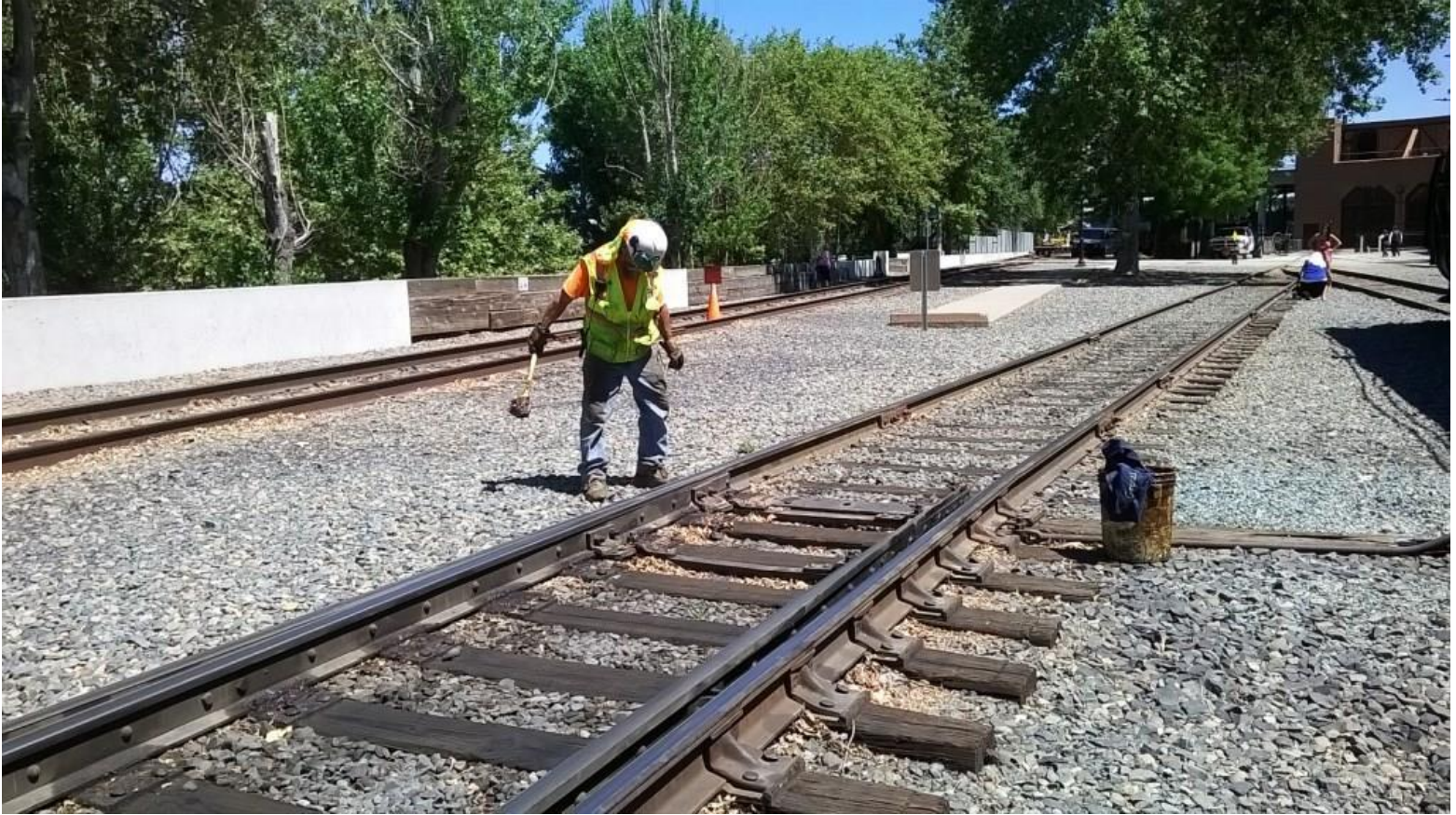
Joe greases the switch with that lovely substance, switch-grease – where's Weston when we need him?
