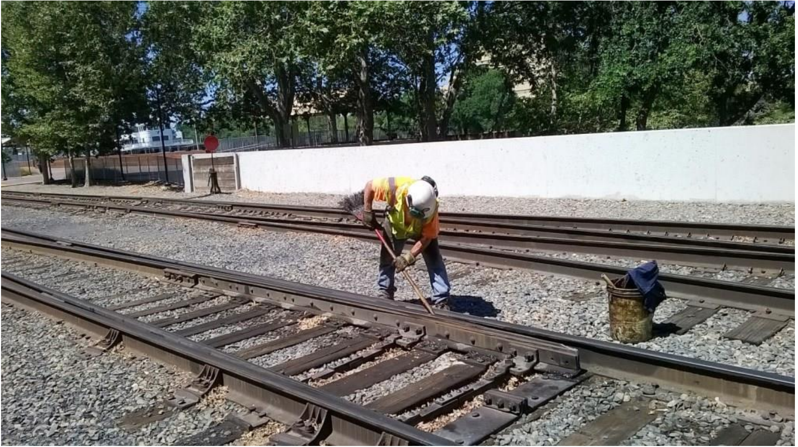
After servicing Switch No. 6, Joe and Heather figured they might as well clean up Switch No. 5 while they were there
