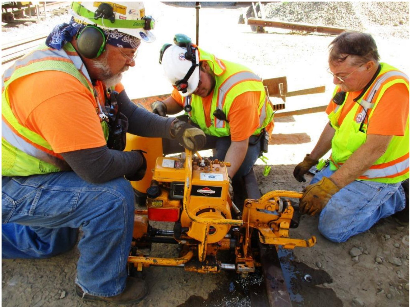
With the first hole drilled, Mike F., Chris, and Mike H. reposition the rail-drill for the next cut
