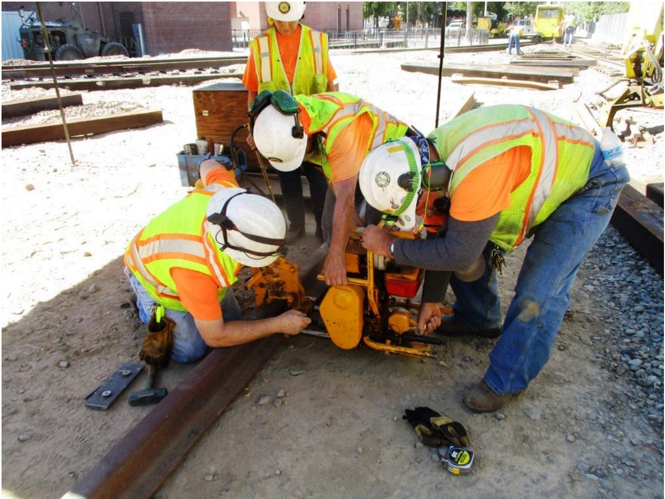
Mike H., Joe, and Mike F. precisely place the rail-drill to cut bolt holes for the heel-block on what will become the diverging stock-rail
