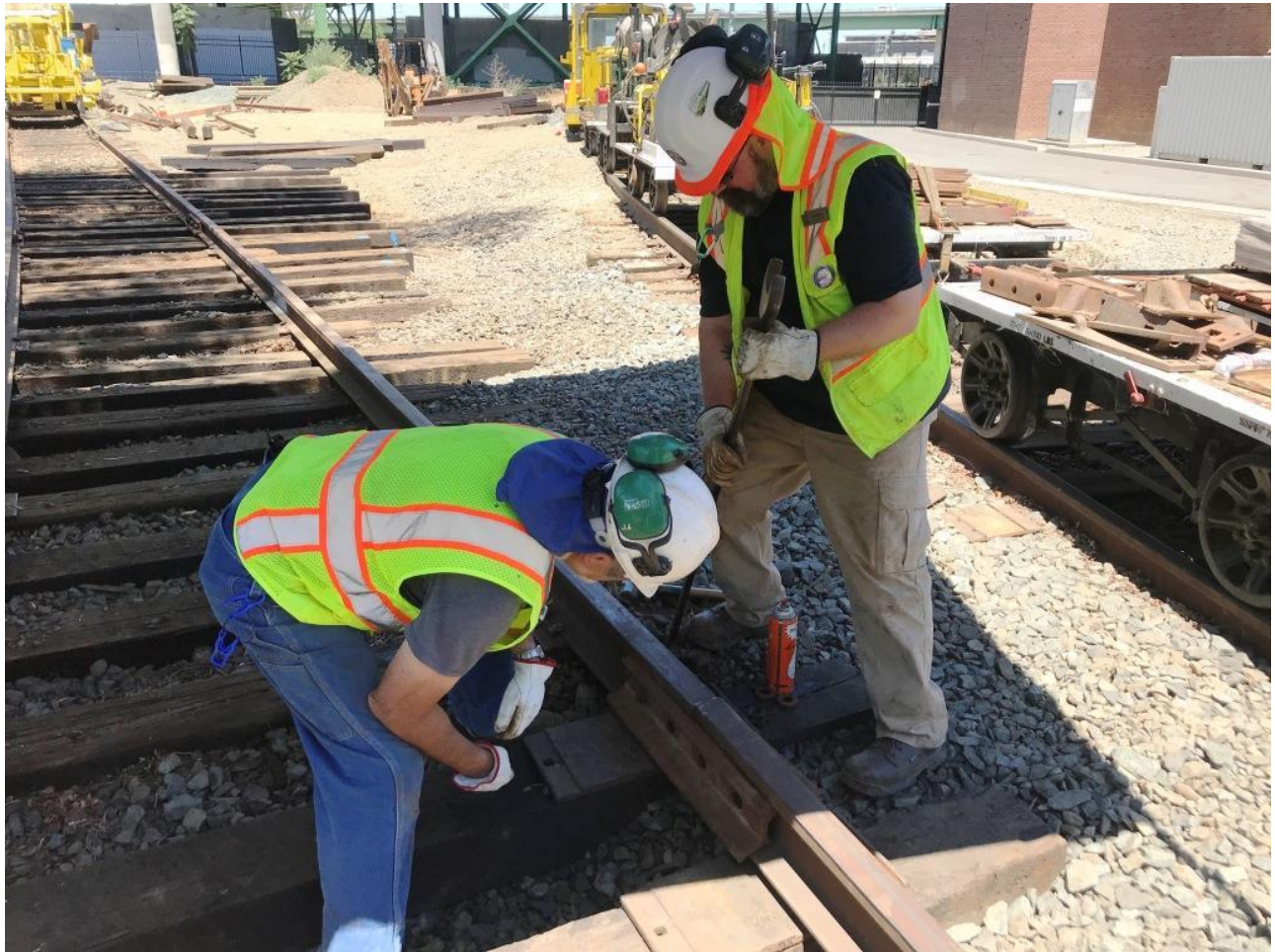
Ed and DJ tighten the bolts on a joint-bar they installed as temporary measure to maintain continuity in the track
