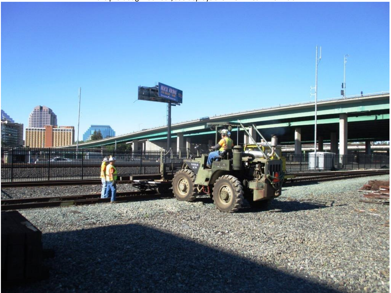
With the Kalamazoo and flatcar spotted near the Boiler Shop, Mike F., on Big Green, loads the 15-foot ties
