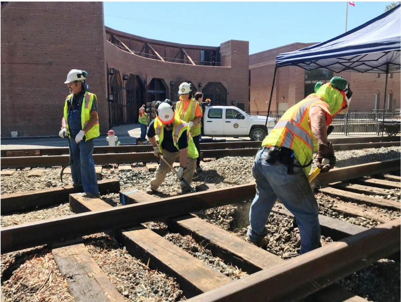
With the 8-foot tie removed, DJ and Joe become the human scarifier and dig-out the crib
