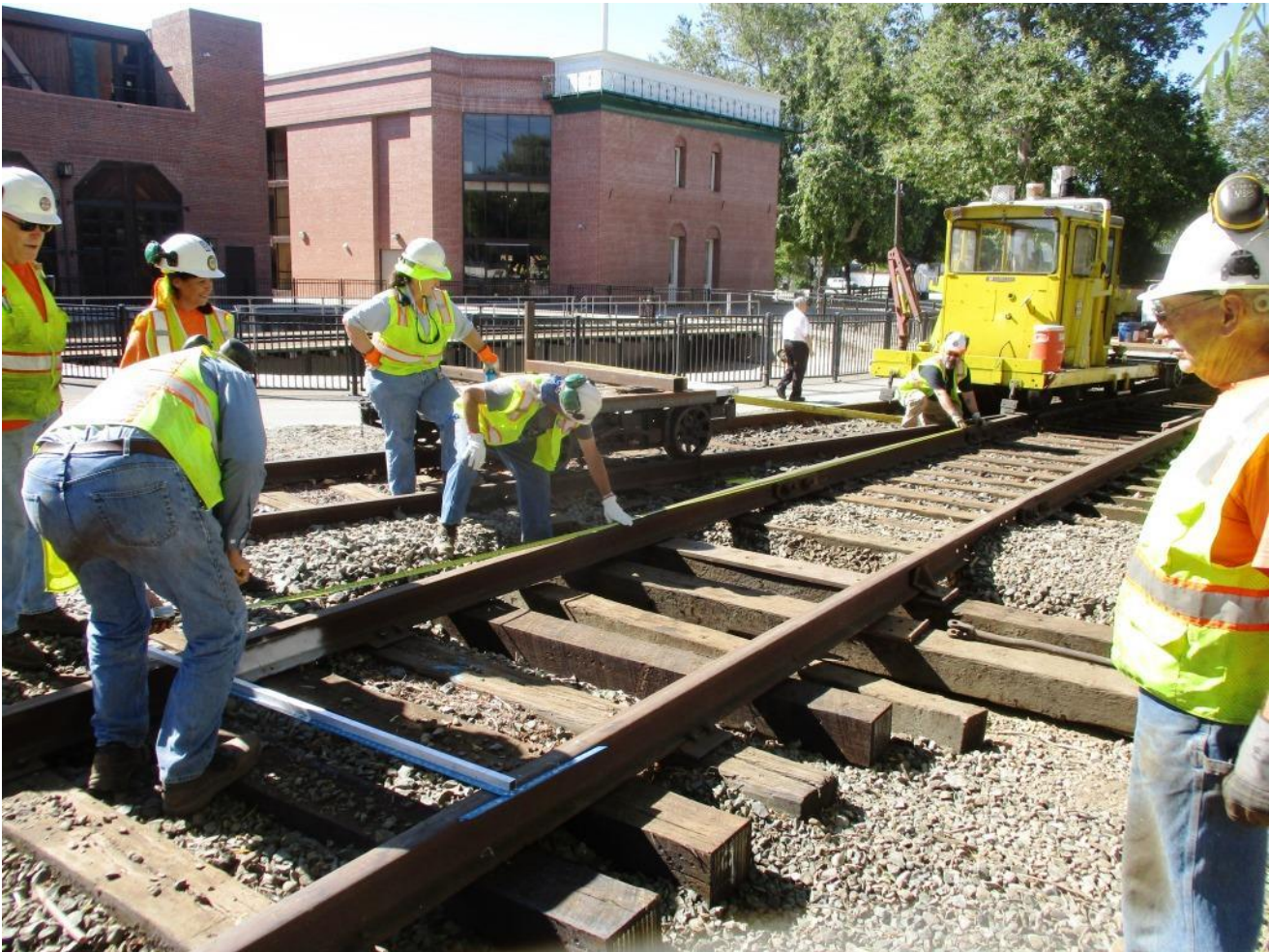
Measure five times, cut once – the Team re-measures all the markings for where the bolt-holes are to be drilled – just to make sure
