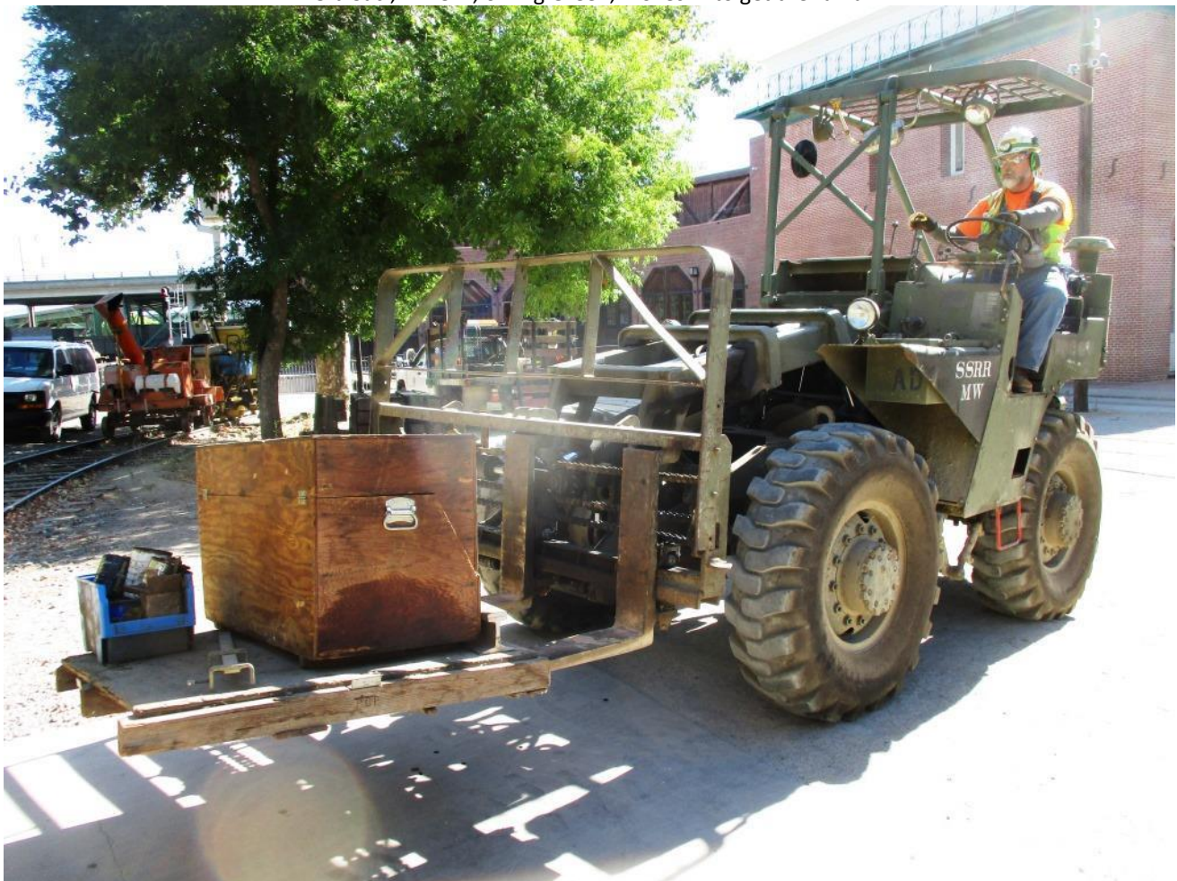
With the rail-drill and accoutrements on Big Green's forks, Mike F. carries it to the work-site
