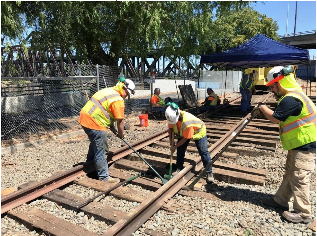
Chris and DJ nip-up the rail as Pam uses a sledge hammer to knock-out the tie place on the next tie slated for removal
