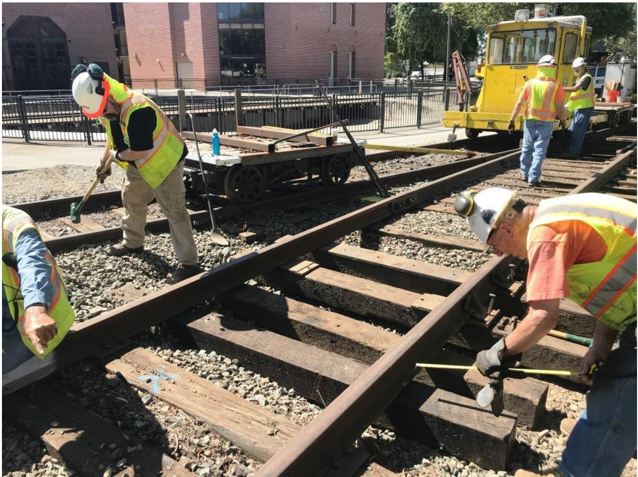
DJ and Clem use a sledge hammer and tape-measurer for precision placement of a 9-foot tie
