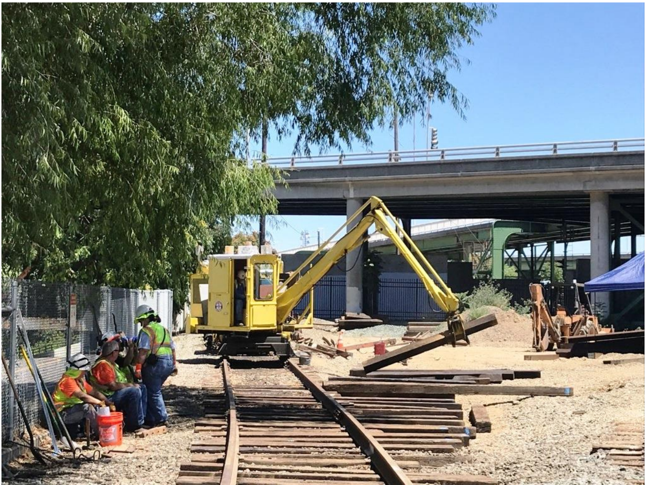
Alan fires-up the tie-crane to move the big ties into position
