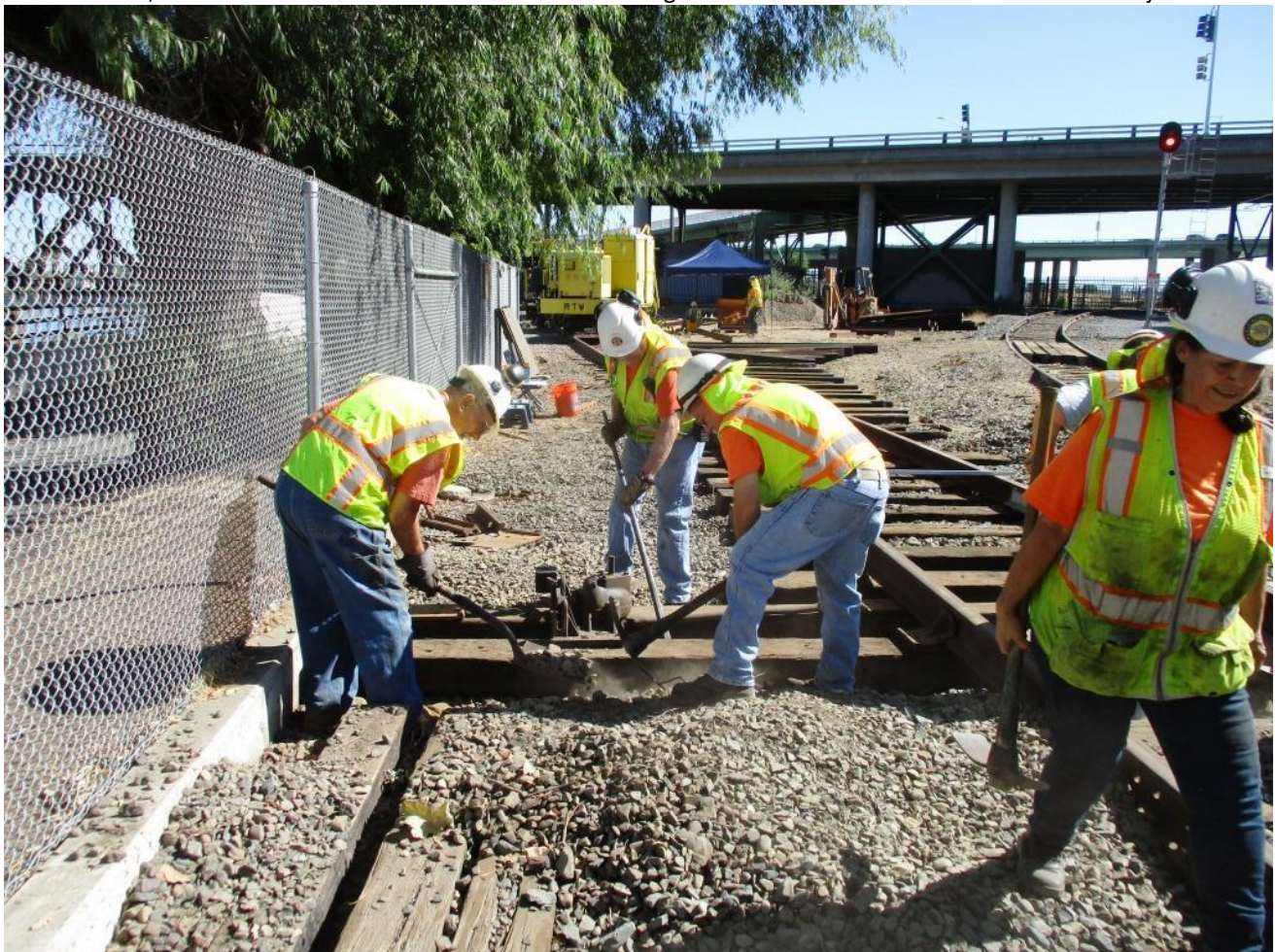
Clem, Bill, and Mike H. remove dirt and debris from the south side of the head-block so it can be moved to a correct position
