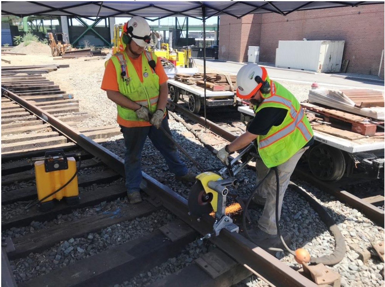
With all 15 holes now drilled, DJ starts cutting the rail with the rail-saw as Chris uses a shovel to shield the sparks
