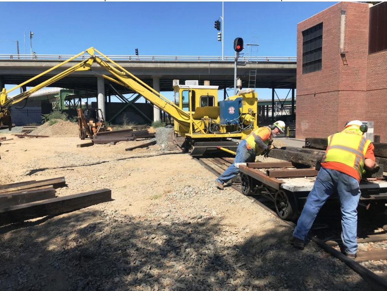
As Alan in the tie-crane cleans up the job-site by picking-up the dead-ties strewn about, Mike F. and Bill arrange them on the flatcar
