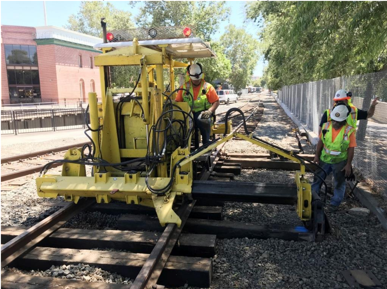
Rather than doing it by hand, Chris uses the Jackson 125 tie-exchanger to pull the next series of ties
